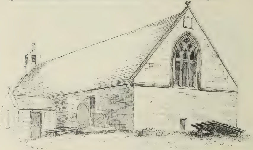
FIG. 1608.—Walston Church. View from South-West.
